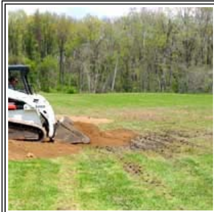
This hastily built sports field was full of bumps and hollows that created an uneven, muddy and unsafe playing surface. Jim Puhalla used his 8-step process to correct the surface defects.
