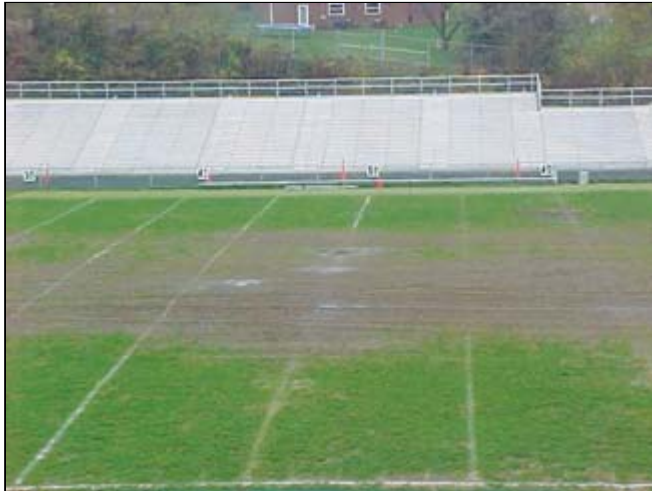
If your football field looks like this one at Indian Creek High School, Wintersville Ohio, it's time for some major repair.
